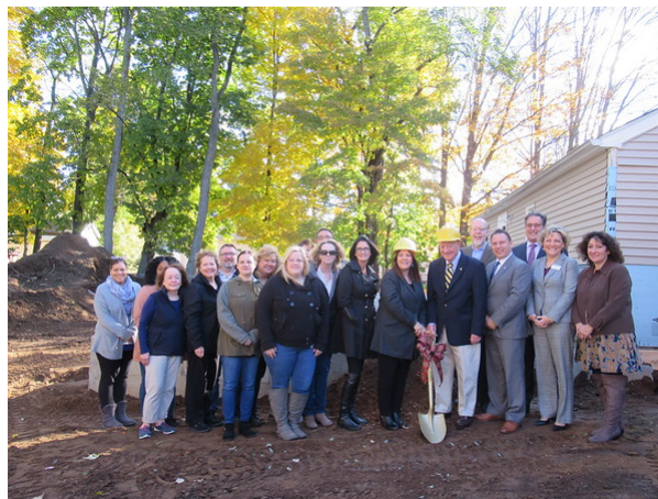
Photo by Susan Corica The ARC of Southington held a groundbreaking Tuesday morning for its new 18,000 square foot addition at its 201 West Main St., Plantsville, location.
