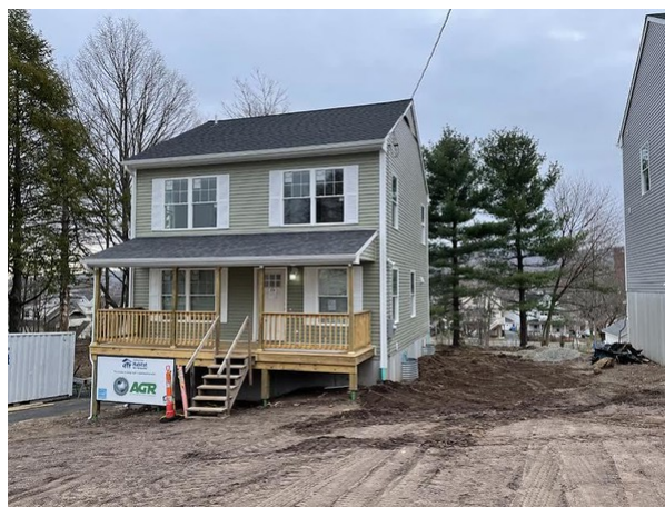
The Bristol homes under construction -Habitat for Humanity
